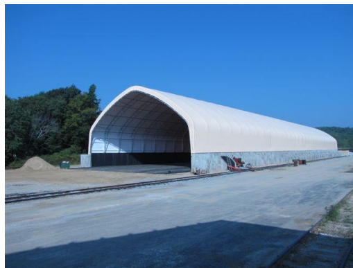
Figure 30 New Mass Central Salt Shed Near Palmer, MA
