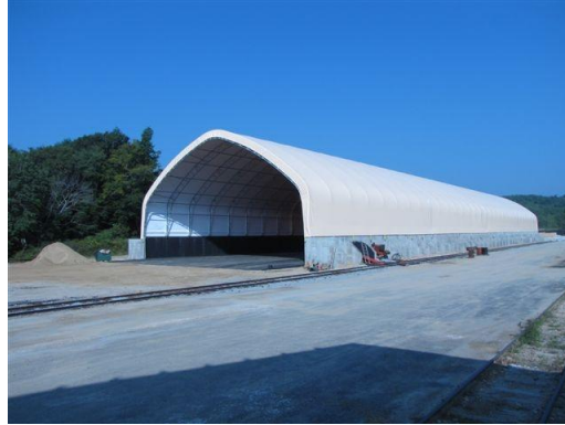
Figure 21 New Mass Central Salt Shed Near Palmer MA.
